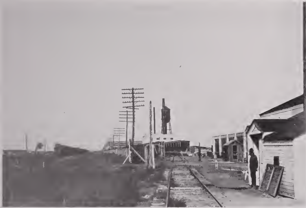
SOUTHEASTERN CORNER PLANT Showing Side Track Entrance
